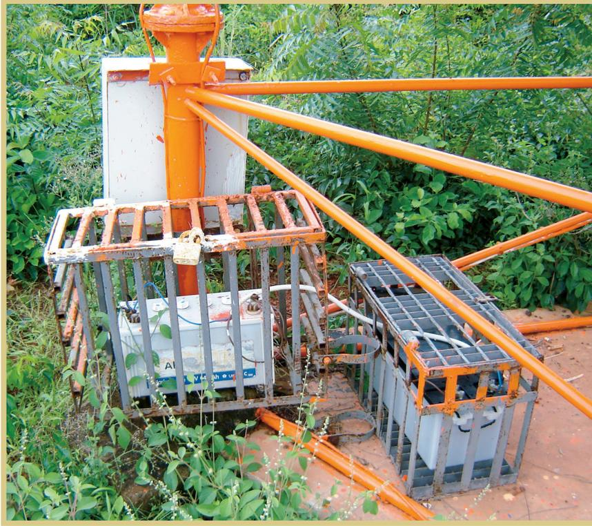
**Figure 3.** A battery in a locked cage in Ghana. Heat dissipates better from the battery in a cage than in a lockbox.
