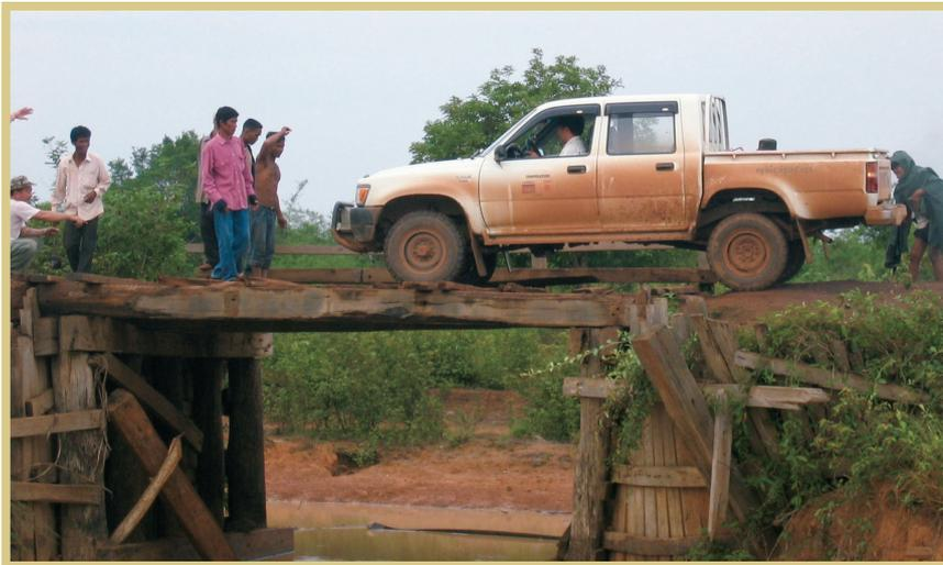
**Figure 2.** This pickup truck was stuck on a bridge in Cambodia that heavy rainfall had damaged.
