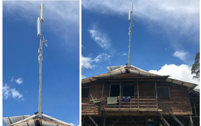
Figure 1: Tower installed on the local school’s roof, reusing existing infrastructure. This CoLTE site is able to cover the entire community from a single location.
