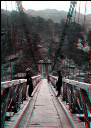
Teesta suspension bridge-Darjeeling, India
