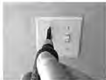
Removing the cover plate, then removing and swapping the switches.
