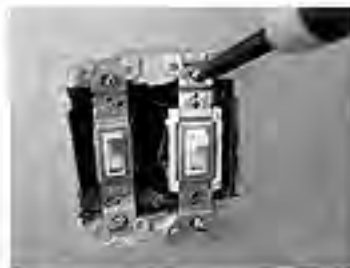
Removing the cover plate, then removing and swapping the switches.
