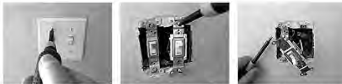
Removing the cover plate, then removing and swapping the switches.
