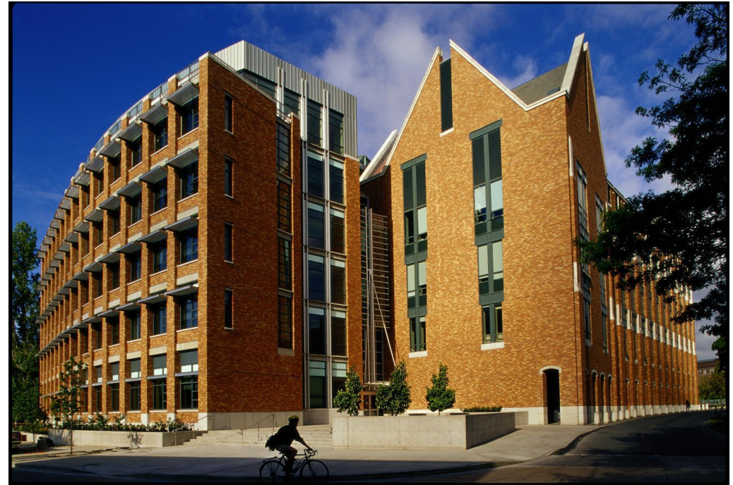
Paul G. Allen Center by LMN Architects
