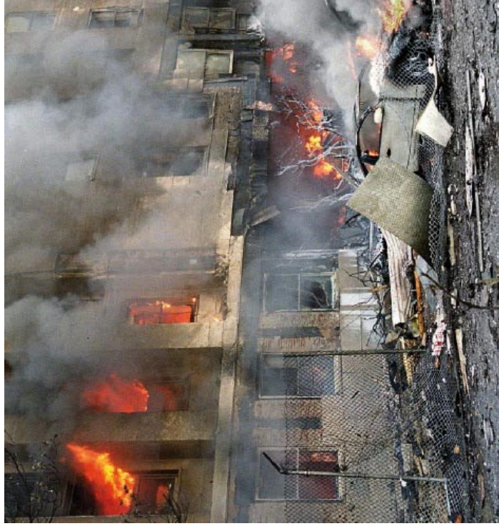
Pentagon on fire and partially destroyed following the crash of American Airlines Flight 77
