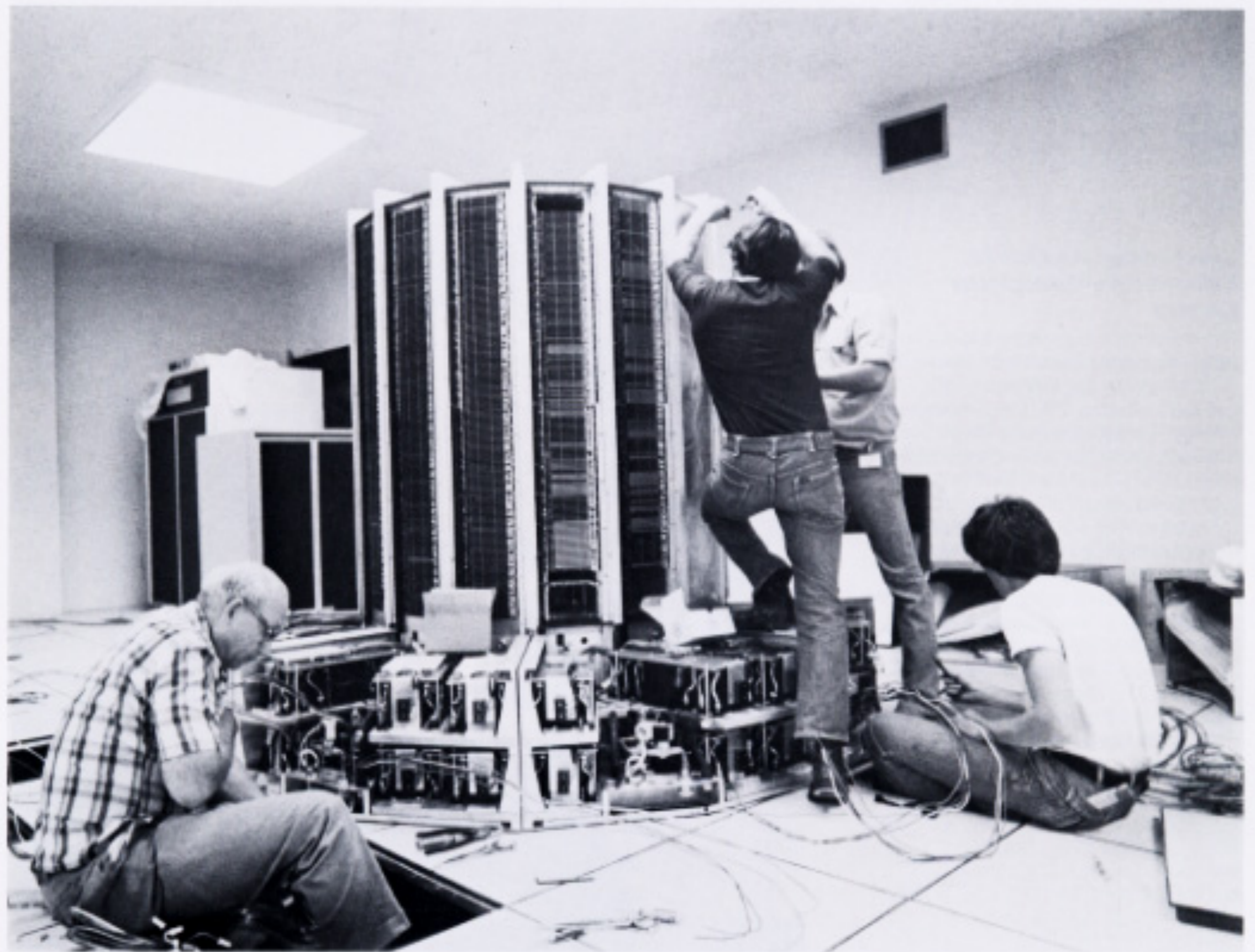
Printed circuit boards and power supply components are exposed as engineers install the CRAY-1 at UCS
